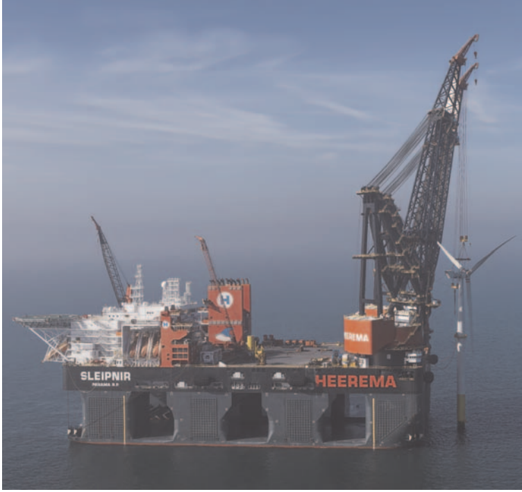
Figure 1. Semi-submersible crane vessel (HMC-Sleipnir) performing a floating offshore installation of an OWT tower [1].
